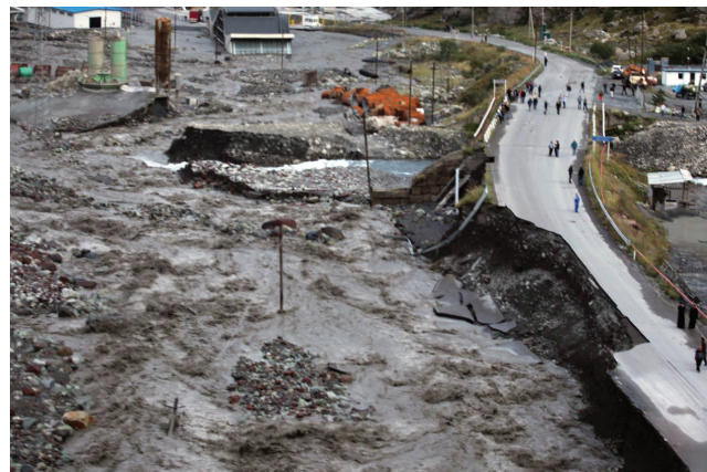
Photo N9 Flood in Dariali gorge
