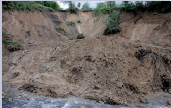
Photo N6 Landslide in the village of Nabeghlavi, Chokhatauri municipality
