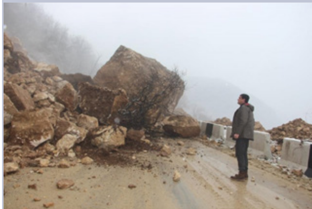
Photo N5 Landslide in Racha
