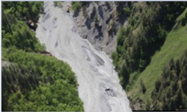
Photo N16 Avalanche on Pshaveli-Abano-Omalo road Photo
